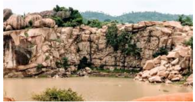
Figure 2: Structural Failure Condition at Jolex Open Pit Mine
