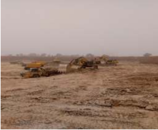
Fig 3: Bulldozer in Operation for Backfilling and Leveling.
