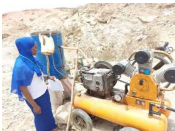
Fig. 15 a: Compressor used in the Area
